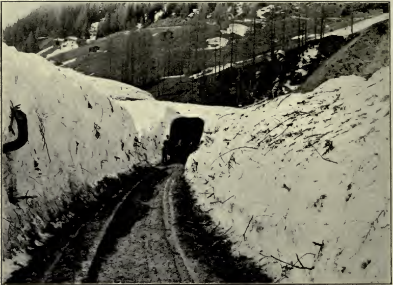
A TUNNEL 300 FEET LONG THROUGH AN AVALANCHE. Tree trunks, etc., can be seen embedded in it.
