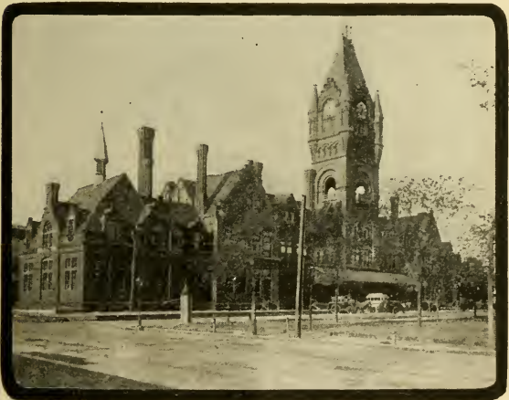
CHICAGO, MILWAUKEE & ST. PAUL R. R. STATION.
