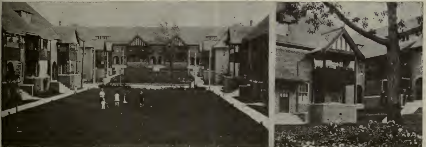
THE architectural problem of the two-family house or cottage flat is met in the Riverdale Courts development of the Toronto Housing Company. "The Lindens," to the left, shows the pleasant effect of double porches and English gables around a grass-covered recreation ground. "The Oaks," on the right, takes advantage of natural grading. Each dwelling has a separate front door, porch and bathroom. Heating is by steam from a central station. Hot water is supplied all the year round.
